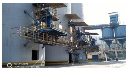
工厂整改后的水泥散装罐车安全平台、护笼 Safety platform and cage for cement bulk tank truck after factory rectification
